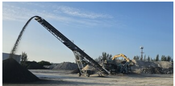
TITAN Recycling Execution (T-Rex) concrete recycling initiative, USA
