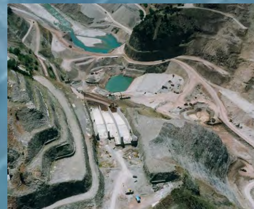
Construction of Sykia Dam
