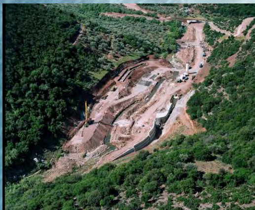
Construction of Peiros-Parapeiros Dam
