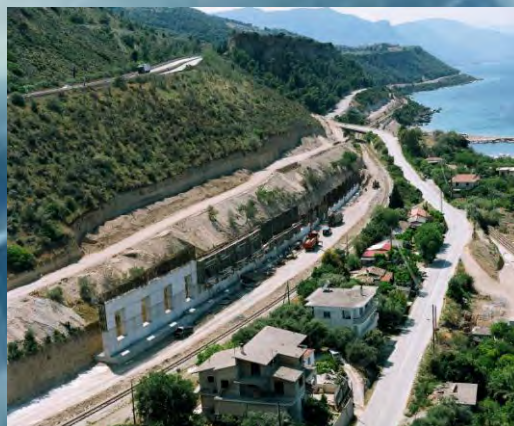
Melissi - Rododafni Railway construction
