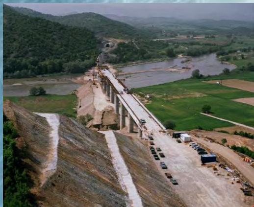
Polykastro – Idomeni rail line construction
